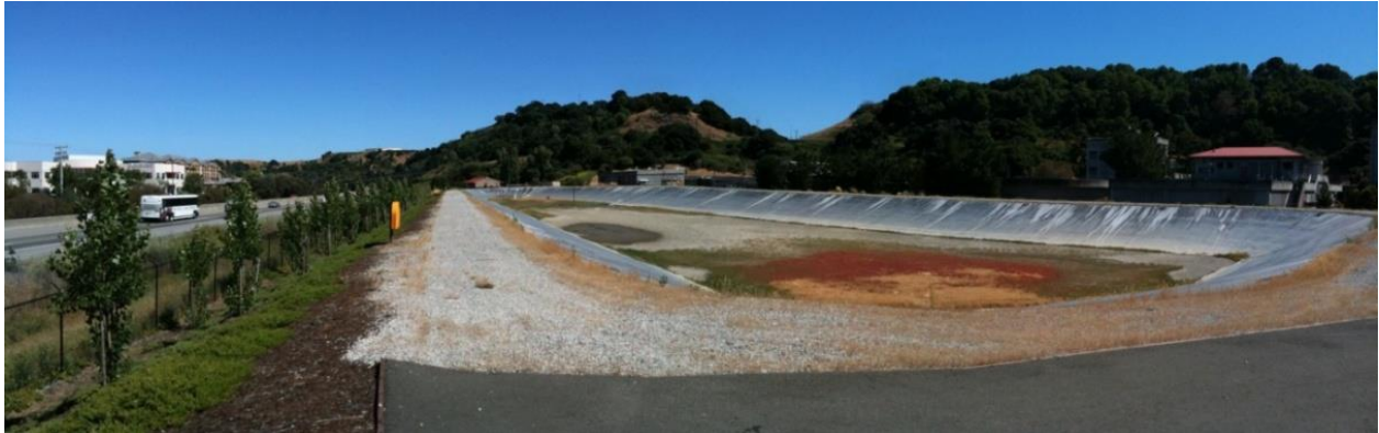
Effluent Storage Pond
