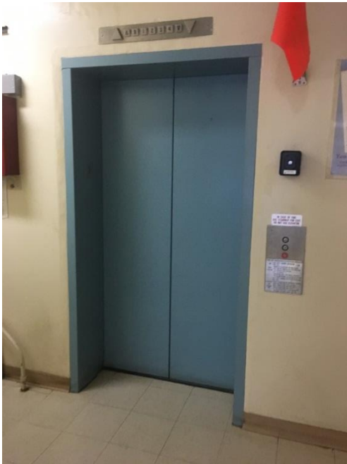
Solids Handling Building Elevator
