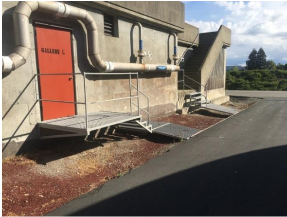
Stair modifications to account for settlement
