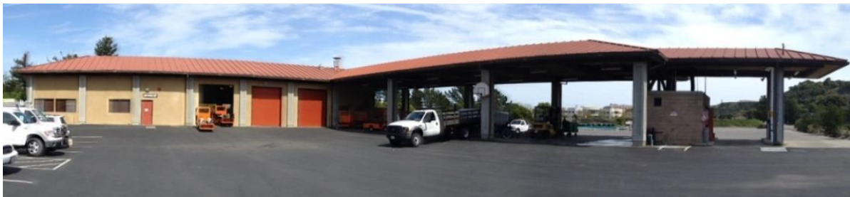
Maintenance Building with standing seam metal roofs
